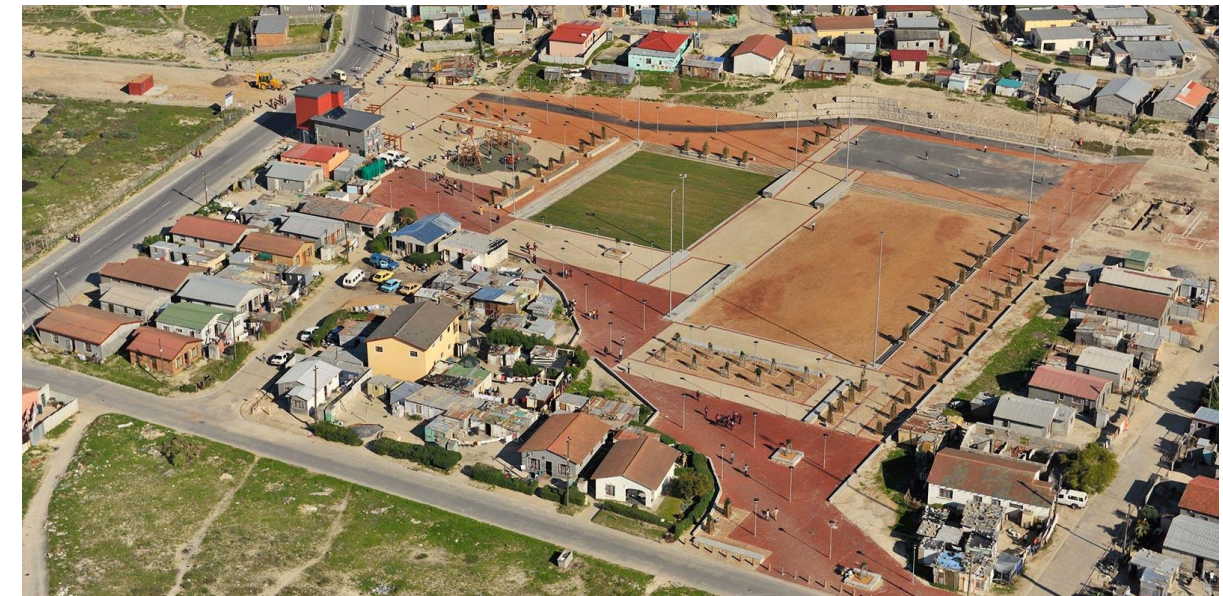
Violence Prevention Through Urban Upgrading (VPUU) safe routes in Harare, Khayelitsha
