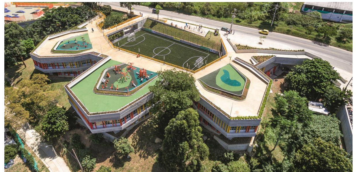
Articulated Life Units (UVA) El Paraiso Precinct in Medellín paired with recreational and cultural facilities such as music rehearsal rooms, auditorium, gym and dance room supporting holistic amenities for communities and connecting to other neighbourhood facilities.
