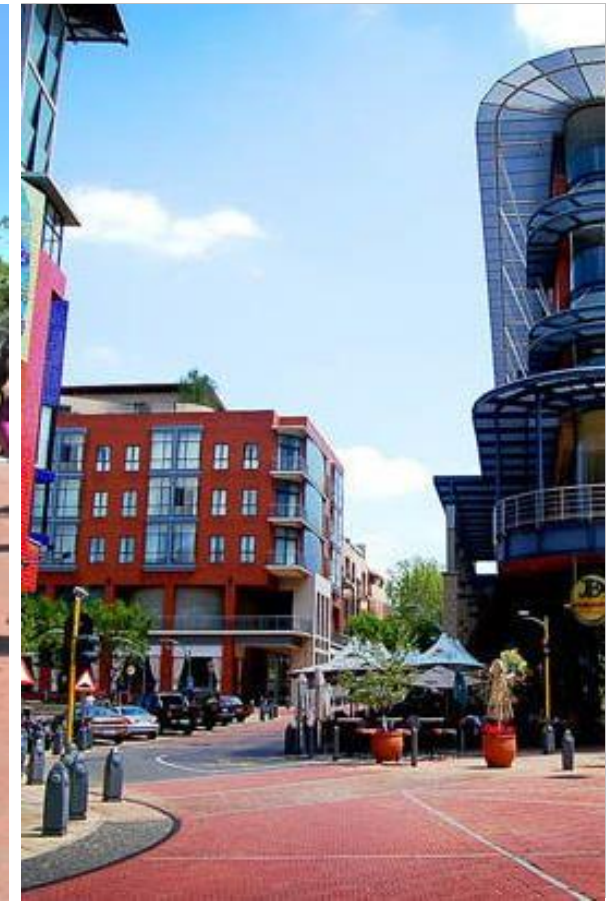
Raised and Paved Intersections at Melrose Arch, Johannesburg.
